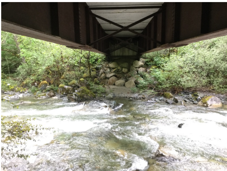
Right Bank Abutment when facing downstream
