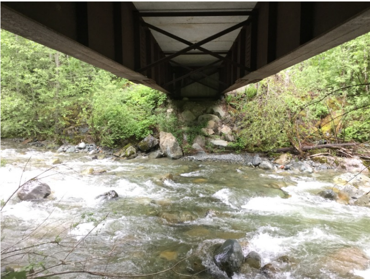
Left Bank Abutment when facing downstream
